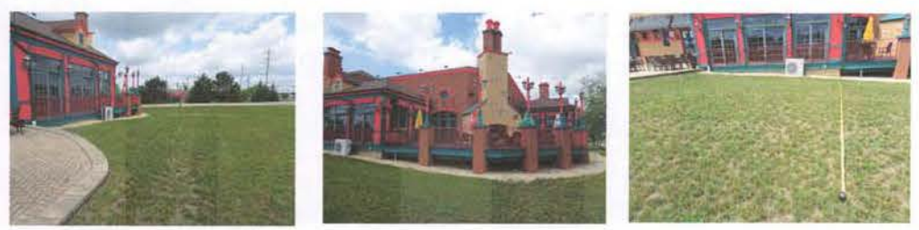
PHOTOS OF EXISTING EASTERN SITE CONDITIONS
