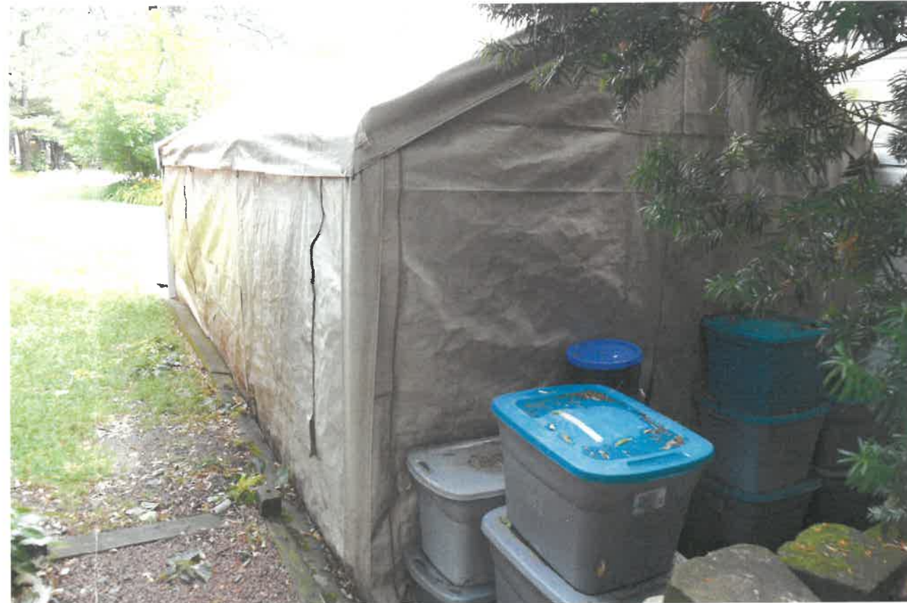
255 INDIAN TR - SW CORNER - LOOKING NORTH EAST
