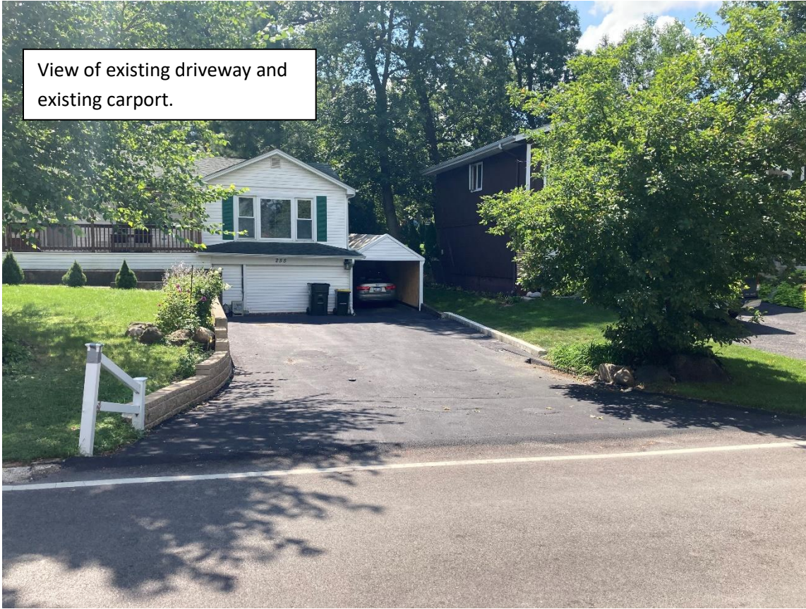
View of existing carport.
