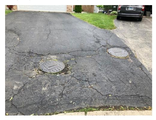
While the manhole on the left is a Village storm sewer, the one on the right is a sanitary sewer. As such, Village staff engaged the Lake in the Hills Sanitary District to assist in the assessment. The first step was to perform a leak dye test, which revealed no leakage and structurally sound manholes. The storm sewer line was televised and showed no defects and was clean. The sanitary sewer line was also televised and showed no defects.
