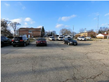
View of police station from south parking lot
