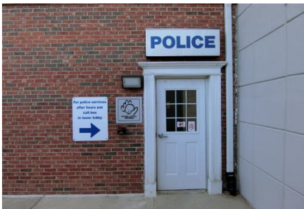
Lower level police station entry and nighttime reception
