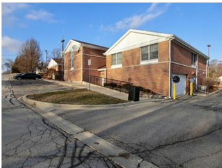
View of police station from southwest
