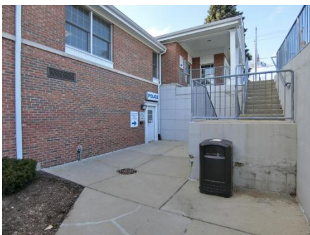
Main and lower level public entries to police station
