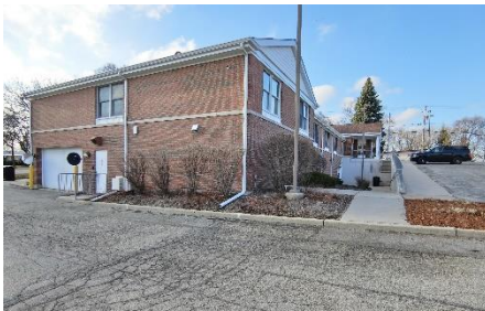
Lower level access – note that it is difficult to see people in this area
