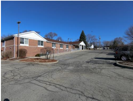
View of police station from southeast
