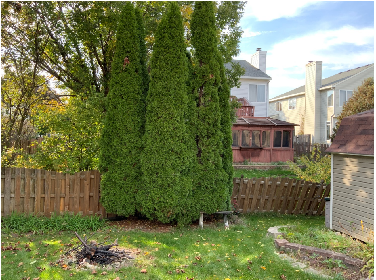
Existing fencing at 261 Wright Drive.
