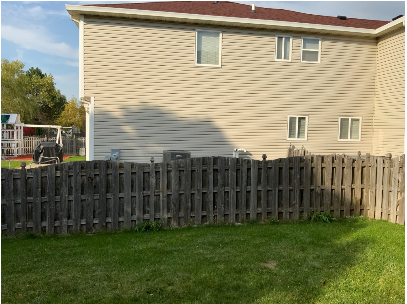
Existing fencing at 261 Wright Drive.
